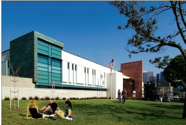
Perkins+Will - LAPD Rampart Police Station Photography: Michael Urbaneck, ArchitecturalShots.com
